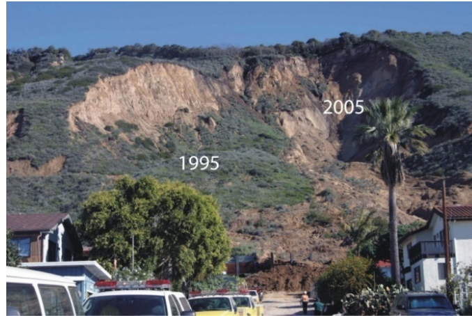
Figure 23. La Conchita following the 2005 landslide. The 2005 landslide reactivated the SE portion of the 1995 landslide. Photograph courtesy United States Geological Survey.
