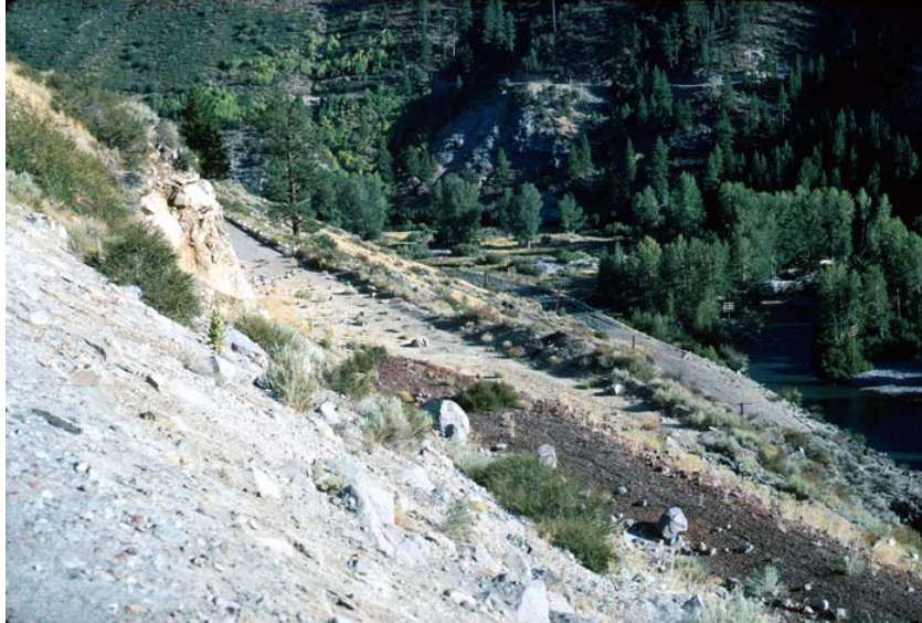
Figure 5. Results of rock fall, Truckee River, California. Large boulders and debris along road were dislodged from steep slope in foreground during an earthquake on September 12, 1966. They fell and bounced down the slope shattering on impact with the road. Photograph by R. Kachadoorian, United States Geological Survey.
