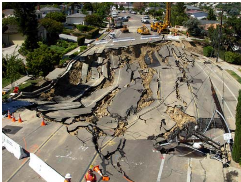
Figure 19. Aerial view of Mount Soledad landslide. Photograph courtesy M. Hart.
