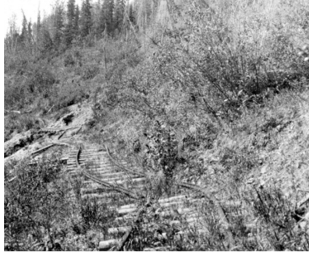
Figure 16. Effects of hillside creep on railroad tracks. Photograph by W.W. Atwood, United States Geological Survey.
