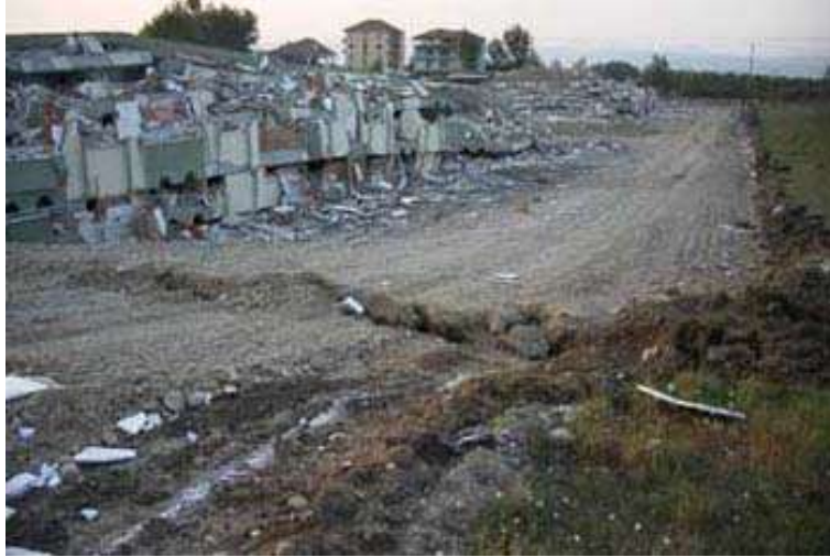
Figure 10. A road is offset in a dextral sense by a surface rupture during the Izit, Turkey 1999 earthquake. The building adjacent to the surface rupture was completely destroyed. Photograph from United State Geological Survey.
