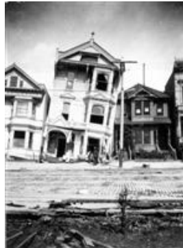
Figure 3. Tilted Victorian in the Mission District following 1906 San Francisco earthquake. Photograph from United States Geological Survey.
